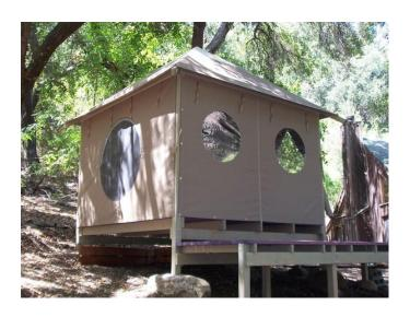
**Tea Room** with a "Moon Window" wall on the left, and a "Port Hole Window" wall on the right, with its central zipper down and the bottom of the wall secured to the edge of the main **Tea Room** deck.
