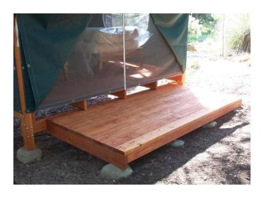
Tea Room with a custom "front porch" attached to the face of its Lower Floor Joist. (Also shows Zippered Entrance wall pinned open over a closed Zippered Screen wall, and a "Moon Window" wall behind one of the new twin beds inside.)
