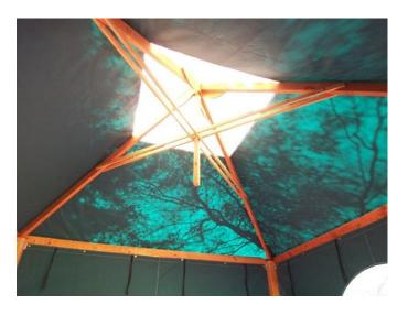
Central "skylights" are standard on all marine fabric roofs for the **Tea Room**. The "Ivory" fabric at the peak of the pyramid-shaped roof admits a gentle glow that fills the whole interior with soft light.
