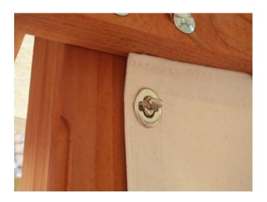
Detail of the fastener used to connect the fabric walls of a **Tea Room** to the structure. Slotted grommets fit over the stem of the fastener, which turns 90° to hold the wall. Two walls can be mounted on each side of the **Tea Room**, a marine fabric wall and a screen wall, to provide for maximum versatility.
